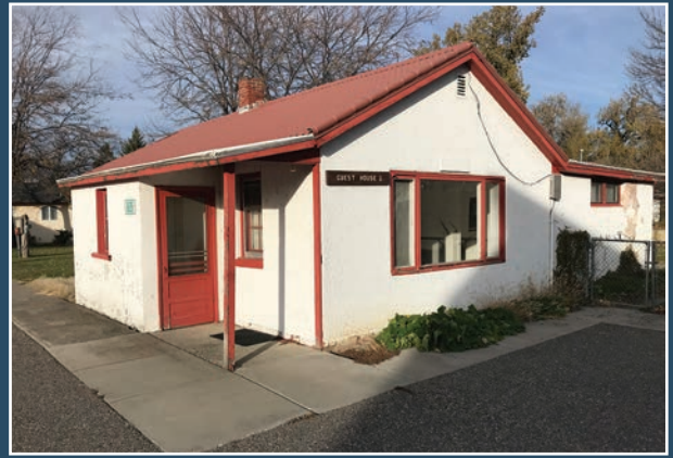
The three bedroom Guest House, another of the original Ranch buildings, provides lodging options for larger families.
