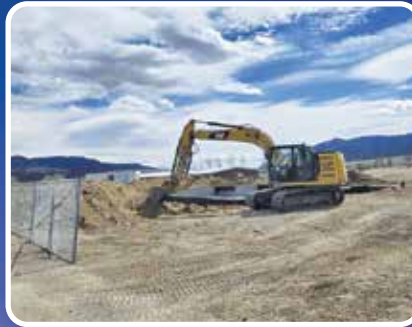
Contractors broke ground on the new home in early spring.
