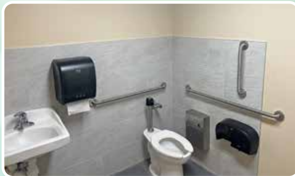
One of the four new bathroom units.
